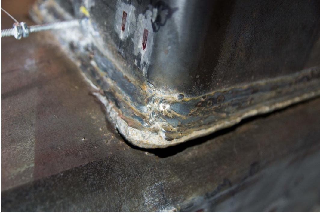
Figure 7.15 Close up of the fracture in the base metal of the column at the toe of the weld in the unmatched connection at the completion of the test
