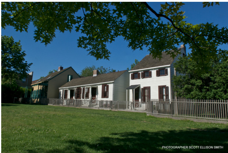
The Weeksville houses arranged along the forgotten Hunterfly Road.
