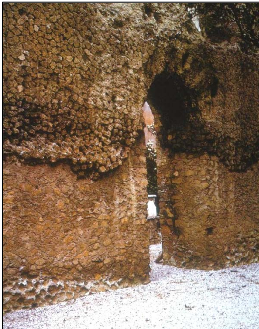
Figure 9: Rome, Testaccio: detail of concrete building with opus incertum facing.
