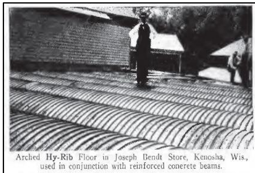
Figure 10. Hy-Rib Concreting.
