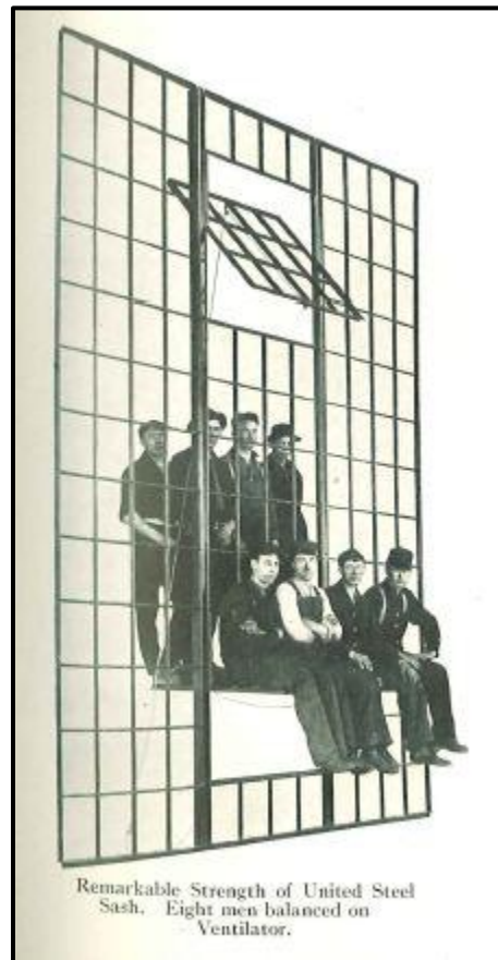
Figure 17. United Steel Sash.
