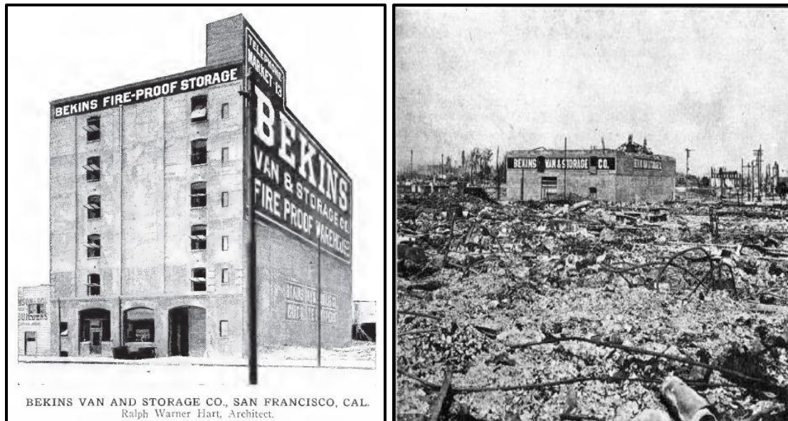
Figure 6. The Van Bekins Building in the aftermath of the 1906 San Francisco Earthquake. Note the Building was only Constructed to the Second Floor at the Time of the Earthquake.
