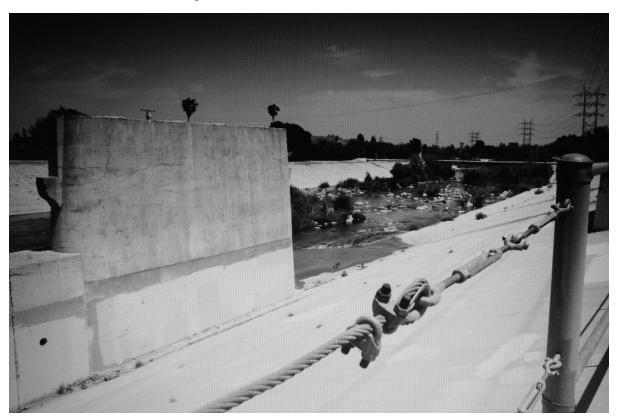
FIG. 31: CONCRETE ENCASEMENT OF THE LOS ANGELES RIVER.
