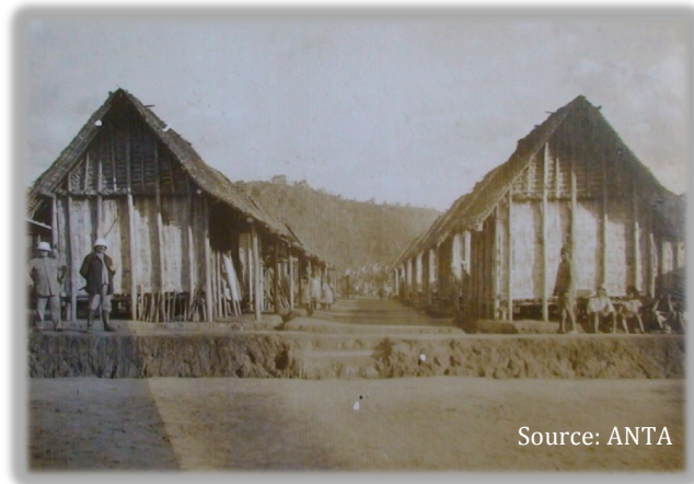
Figure 4 SMOTIG camp barracks at Tolongoina (June 1930)
